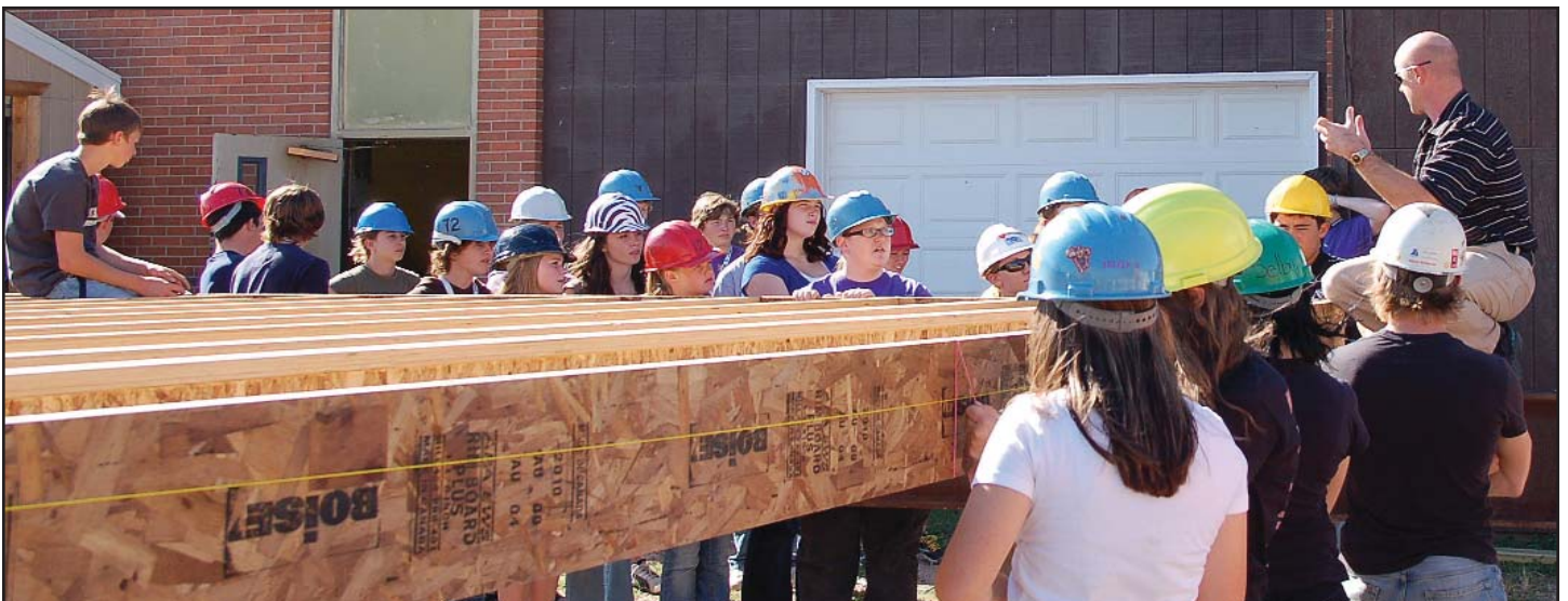
Geometry-in-construction teacher Chad Hedderman, far right, explains to the students the importance of making sure the house is perfectly square before they begin gluing and screwing down the floor. He also reminded the students to utilize their knowledge of geometry in making sure each corner is square.
