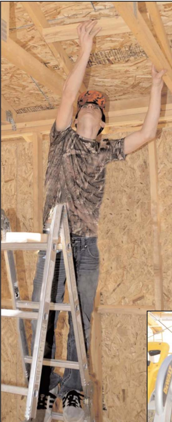
**Above: Alex Voges works on blocking the roof to ensure that it is capable of supporting the weight of a roofer.**
