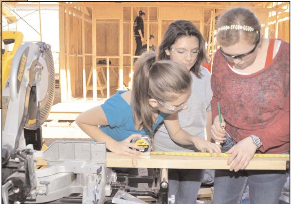
**Right: Cante Permann, Reese Huck and Chyann Cody measure before using the miter saw to make precision cuts for the blocking material.**
