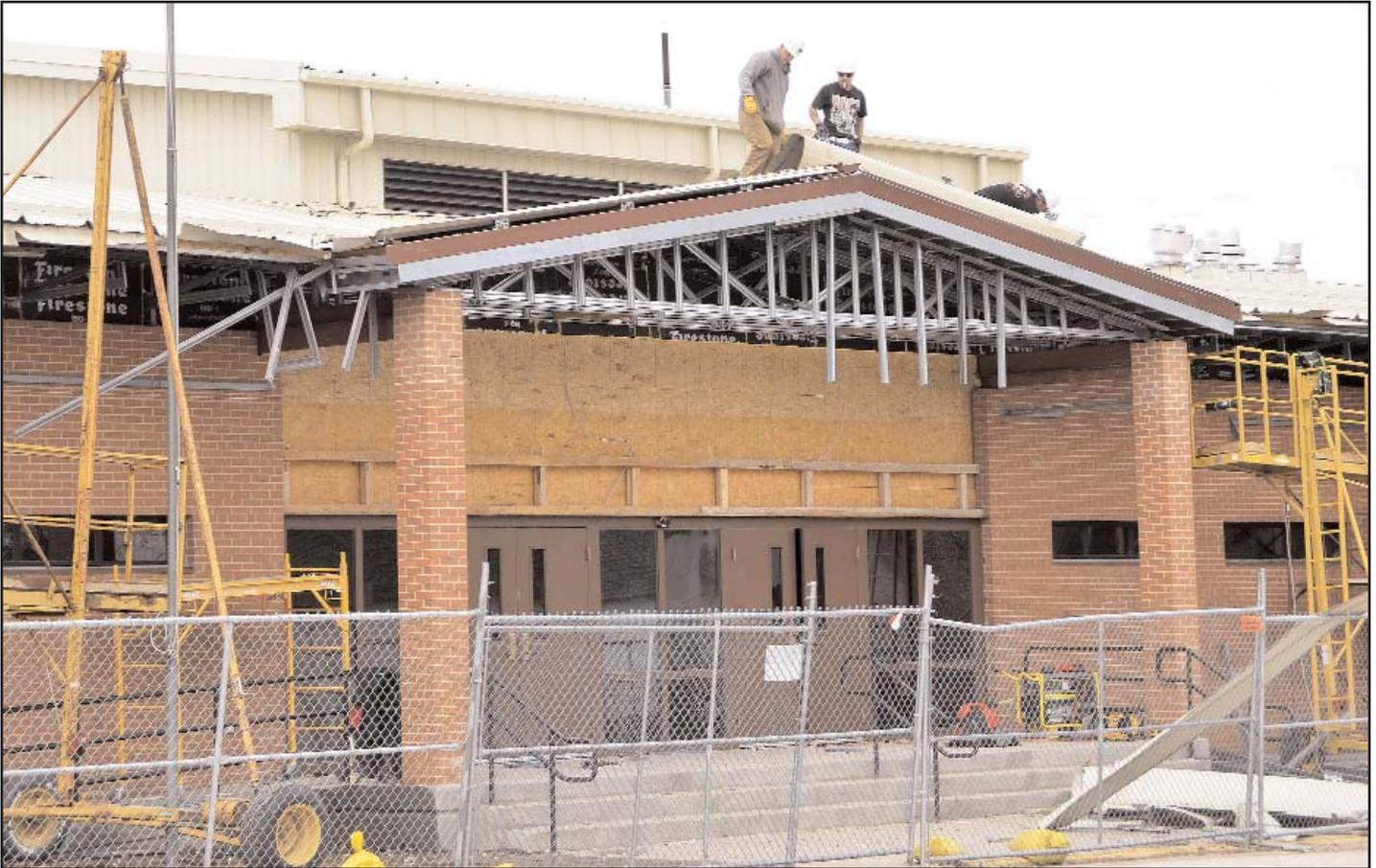
*Ainsworth-Benning workers remove sections of the damaged roof at Sturgis Williams Middle School including multiple layers of oriented strand board and insulation. The roof was then covered with weather proof material until the trusses are delivered and can be installed. (Photo by Kris Hubbard)*
